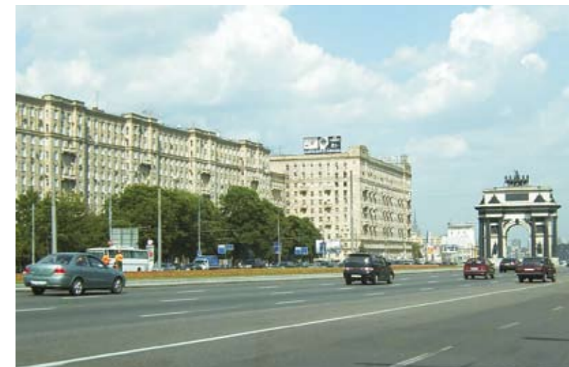
LEG's international office in Moscow is located in a building near the historic city center.
