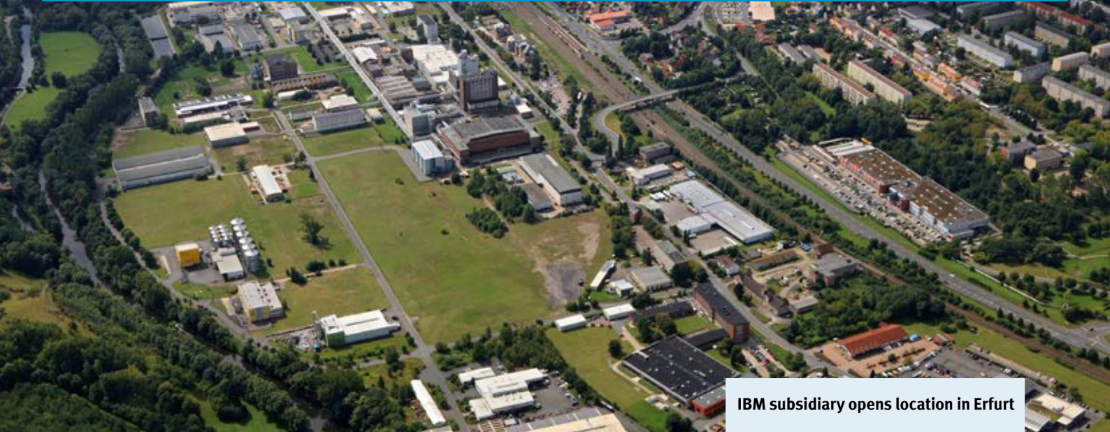
In the Rudolstadt-Schwarza industrial site, the Korean company SungEel HiTech and its partner Samsung C&T Deutschland GmbH will in future strengthen the Thuringian battery cluster with a state-of-the-art recycling plant. Photo: LEG Thüringen; Michael Mehner-Amm/fotoflug.de
